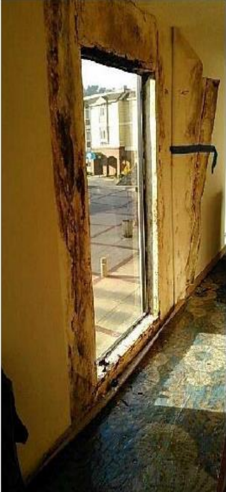
Mold and Decay around windows
