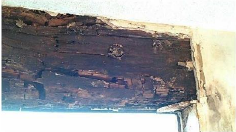
Window Header decay
