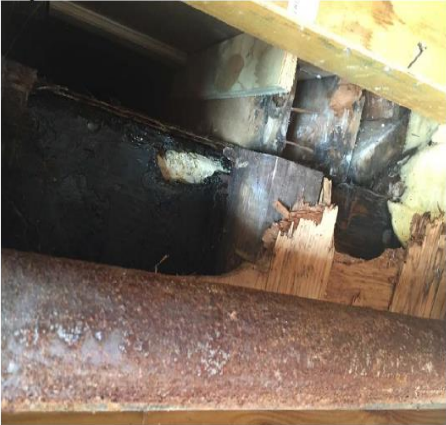
Damage below roof deck
