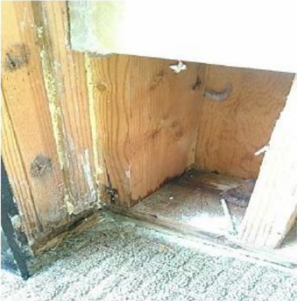
Damage at exterior walls
