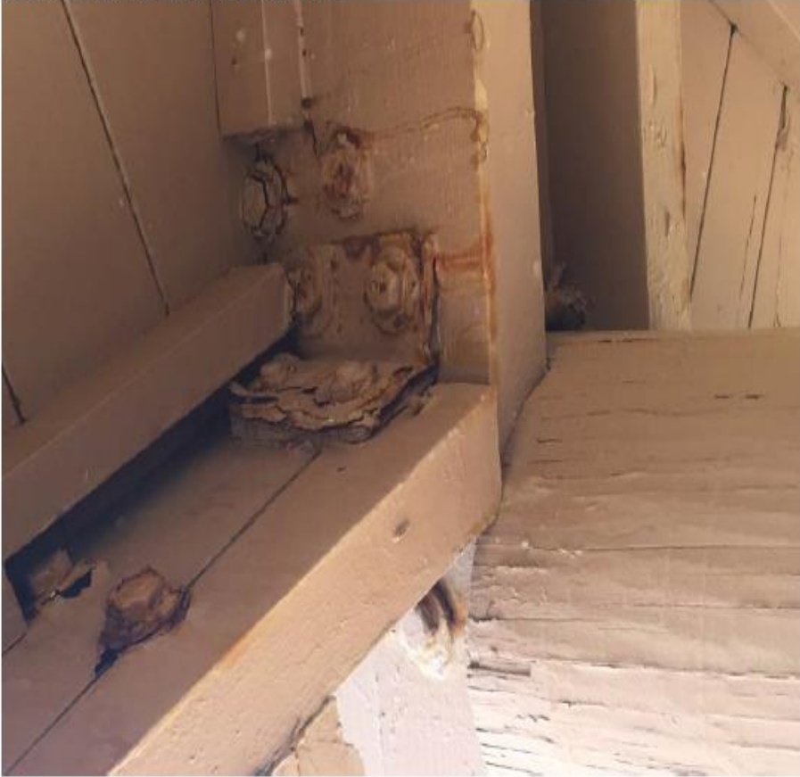
Decayed Deck members and connectors
