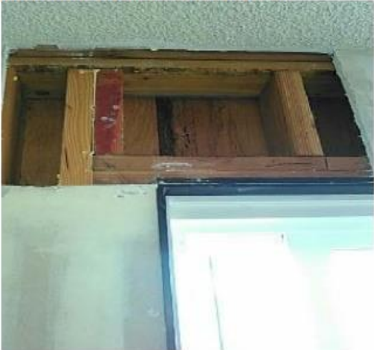
Windows installed without headers above
